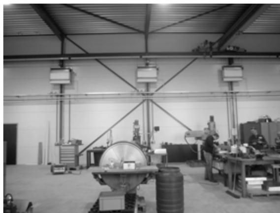
Figure 6: Fiwihex very low temperature heating and cooling device in a machine factory
