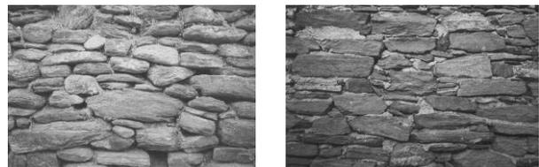
Figure 3: Stone wall construction in Sifnos (a) with local stone and earth mortar and (b) with slate and cement mortar.
