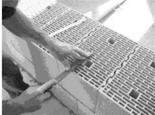
Figure 2: Ziegel walls blocks showing cellular construction [6]
