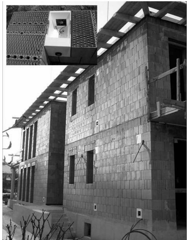
Figure 5: Ventilation equipment of a family house during construction
