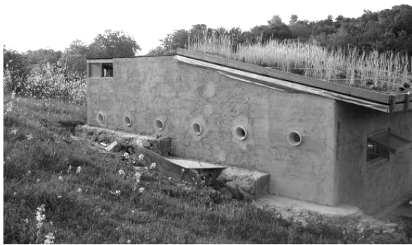
Figure 11: Green Roof of the Tijuana House (north view)
