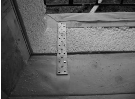
Figure 7: Three layer construction of outer wall, Lidköping
