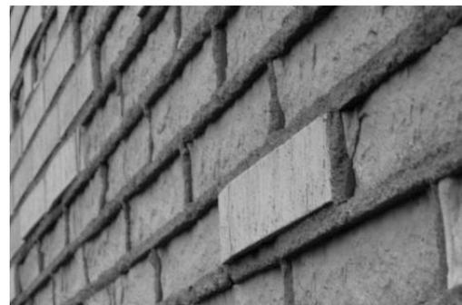
Figure 10: Worn out brick façade, Alingsås
