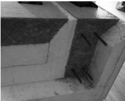
Figure 2: Double L-insulation in ground construction, Värnamo
